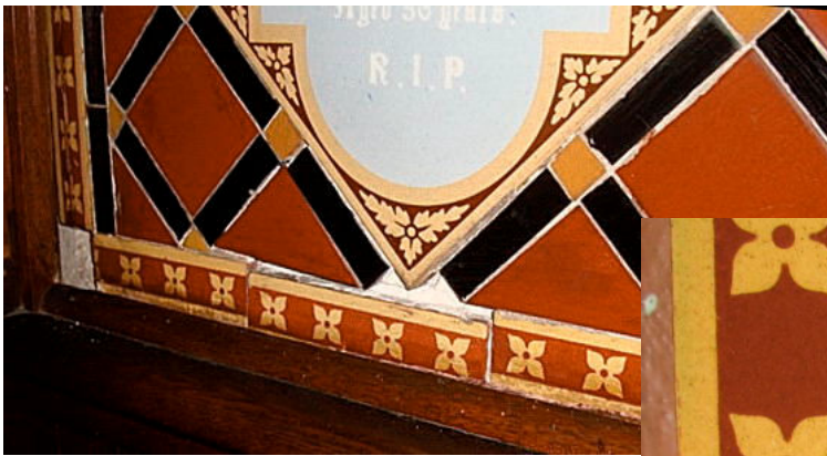
A four-petal corner piece and two triangular mosaic tiles are missing in the photo above. In addition, the central four-petal piece is misaligned. The photo to the right shows a poorly set "extension" to a four-petal tile.
