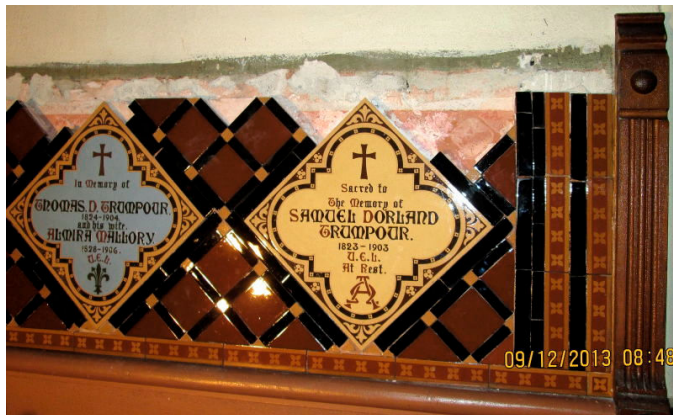
Loose tiles removed from frieze
